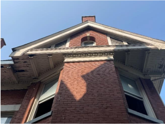
Photo 40: Gabled bay projection, chimney, and rounded arch window, east façade
