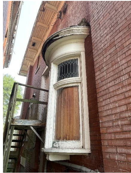
Photo 37: Curved window detail, west façade
