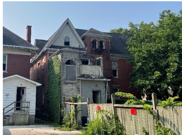
Photo 27: North façade, looking southwest
