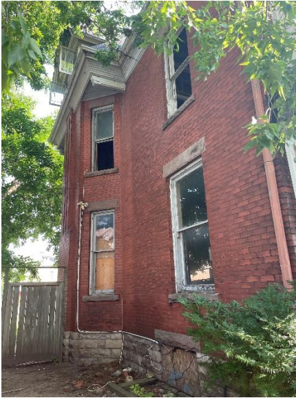
Photo 24: Western façade, looking northeast
