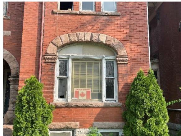
Photo 19: First storey of the eastern bay of the front façade, looking north
