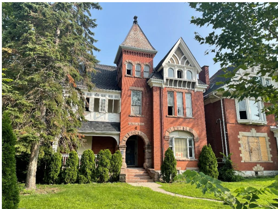
Photo 13: Front (south) façade of 300 Princess Avenue, looking north
