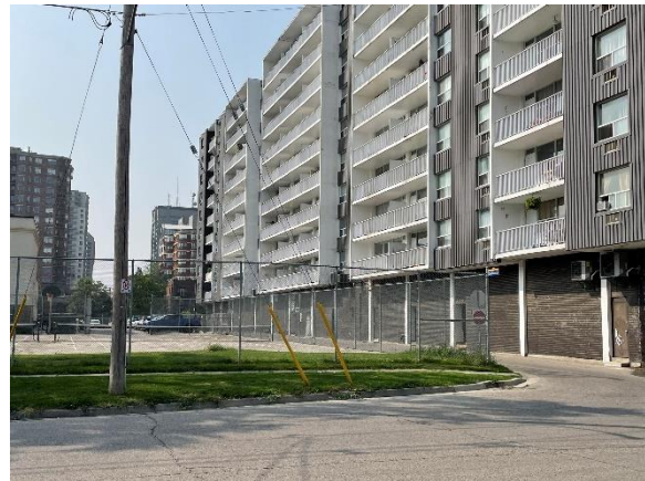
Photo 8: Apartment building west of Study Area, looking south
