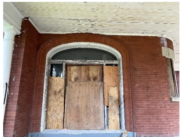
Photo 31: Front entrance door
