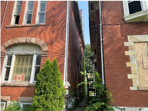
Photo 22: Eastern façade, looking north
