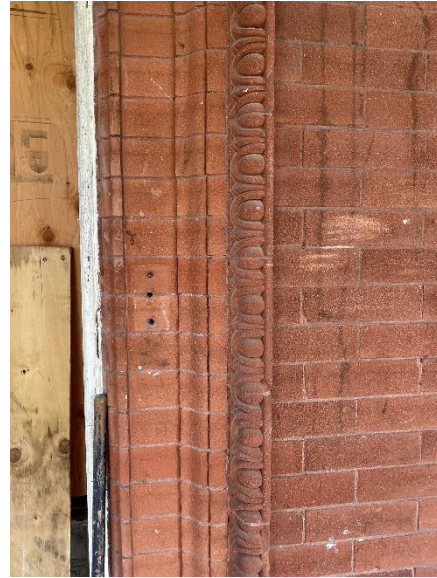
Photo 33: Brickwork surrounding front door
