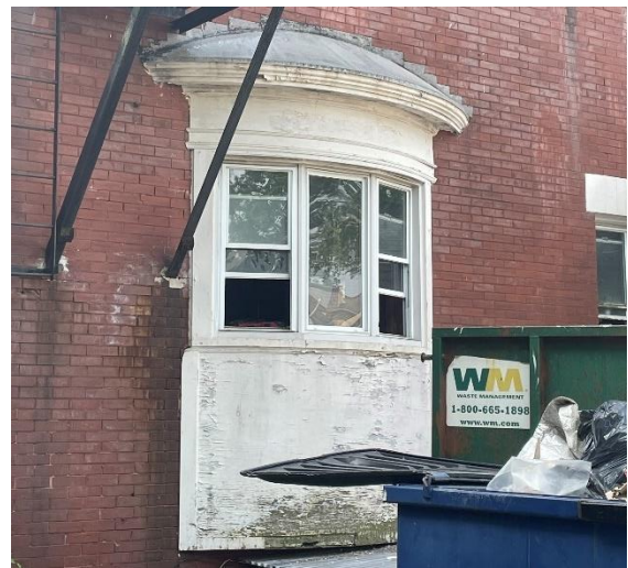
Photo 43: Curved bay window, north façade
