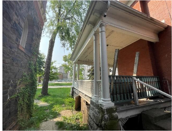
Photo 41: East façade wrap-around porch
