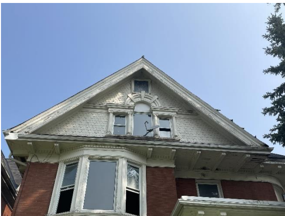
Photo 30: Palladian window on south gable
