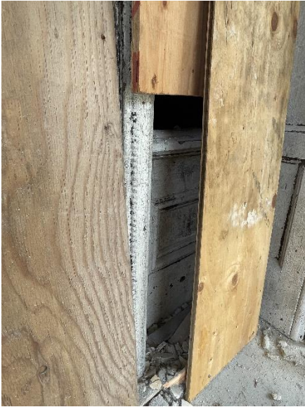
Photo 32: View of wood paneled door beneath plywood covering
