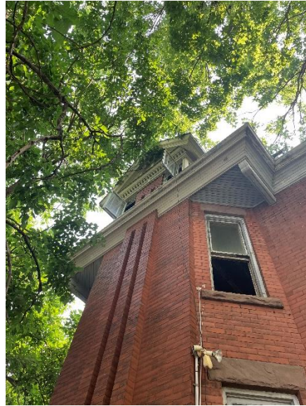
Photo 25: Projecting bay and gable peak on the western façade, looking northeast
