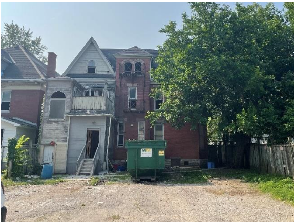
Photo 26: North façade, looking south
