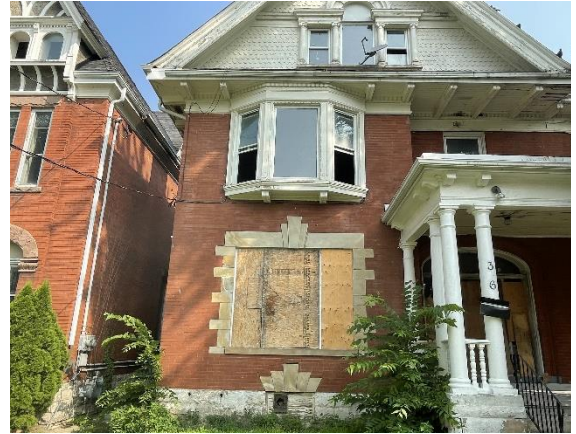
Photo 29: Easternmost bay on south façade
