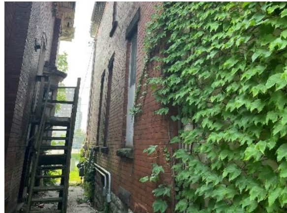
Photo 23: Eastern façade, looking south
