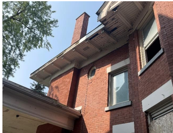
Photo 39: Oval and rectangular windows, east façade
