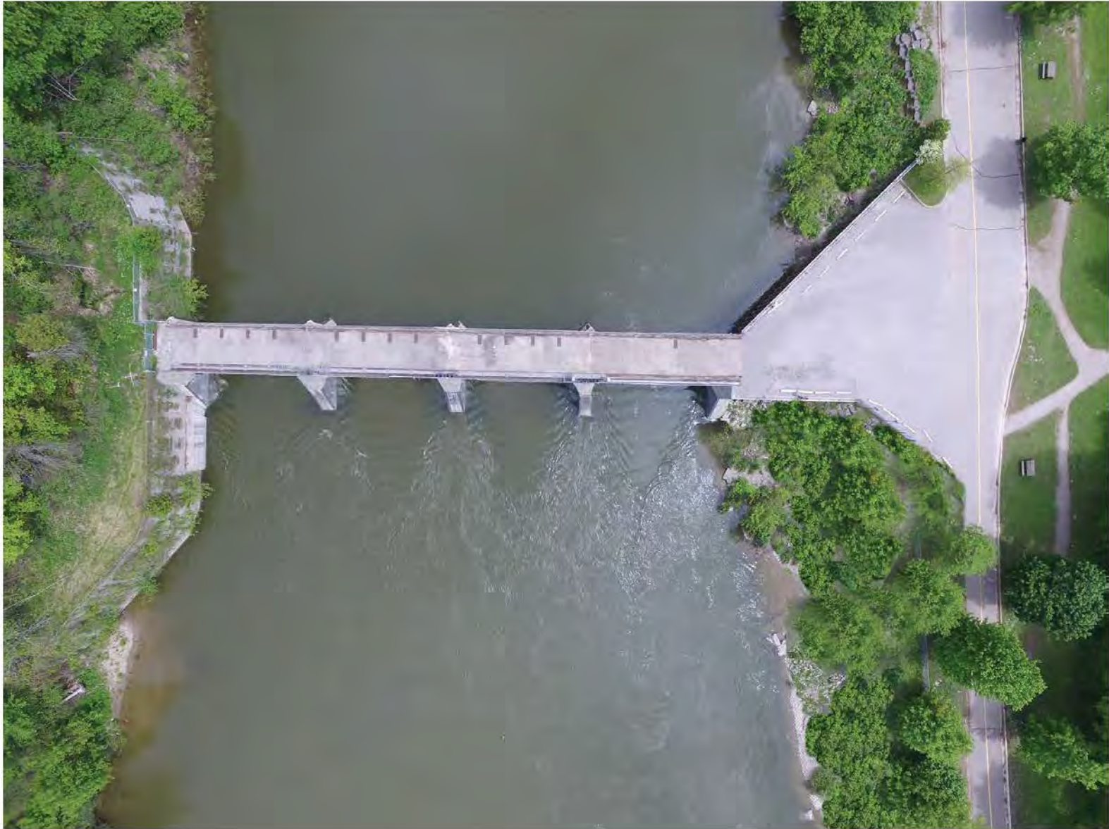
Figure 5-3. Partial Dam Removal Alternative One River EA City of London London, Ontario
