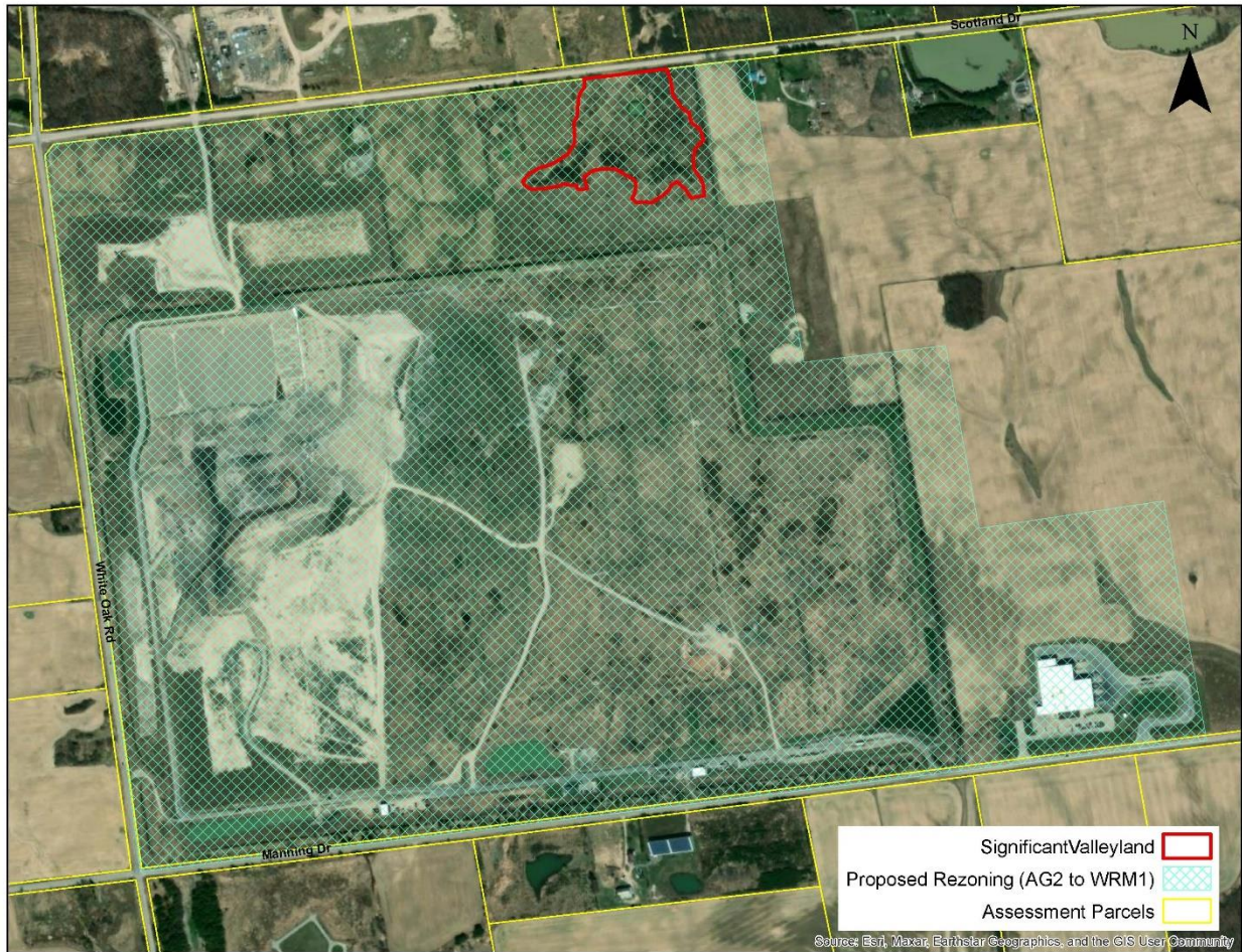
Figure 6 – Image of subject lands illustrating the future areas that will comprise the WRM1 zone and the OS5 zone should the requested zoning amendments be approved
