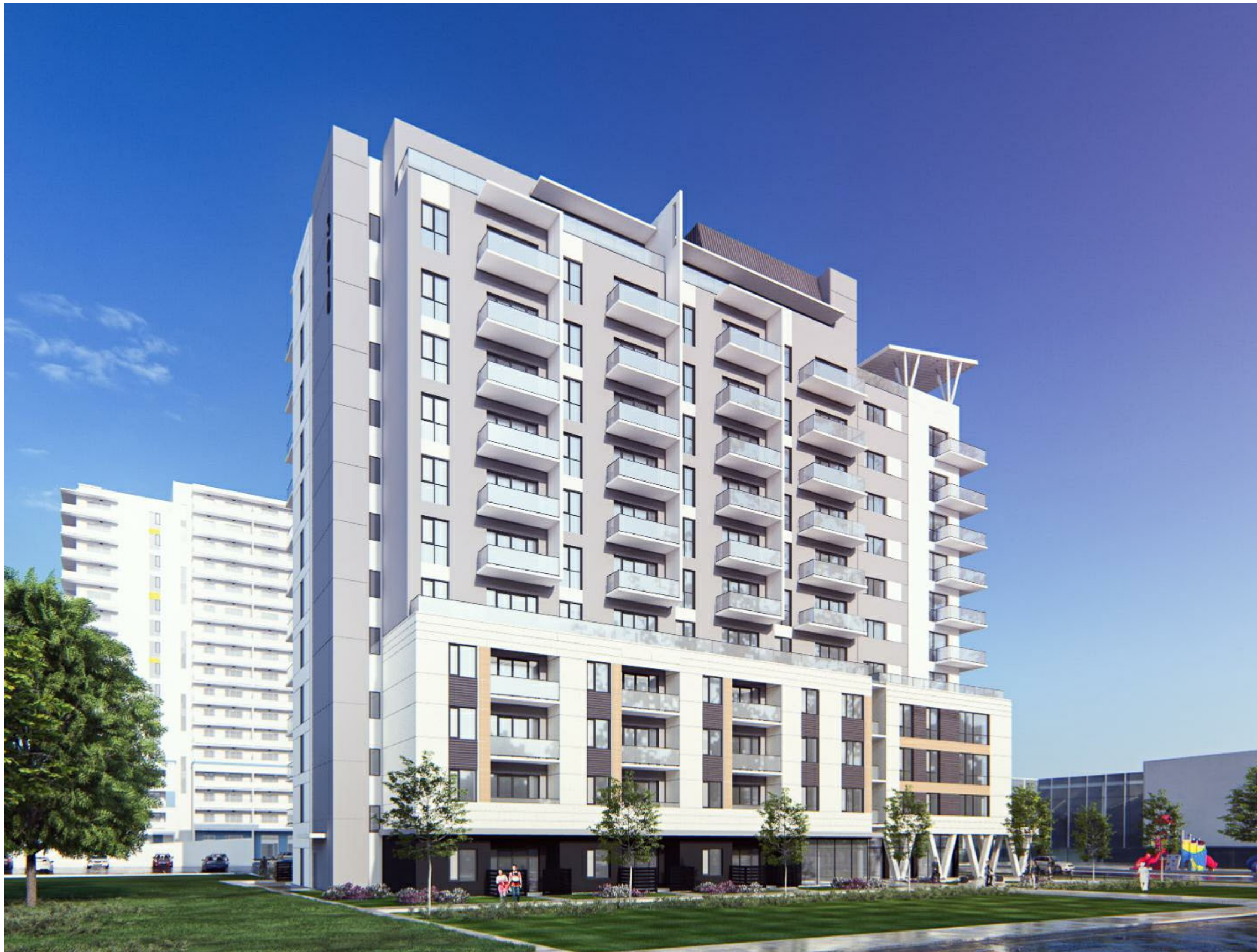
View from Southdale Rd W looking Southwest
