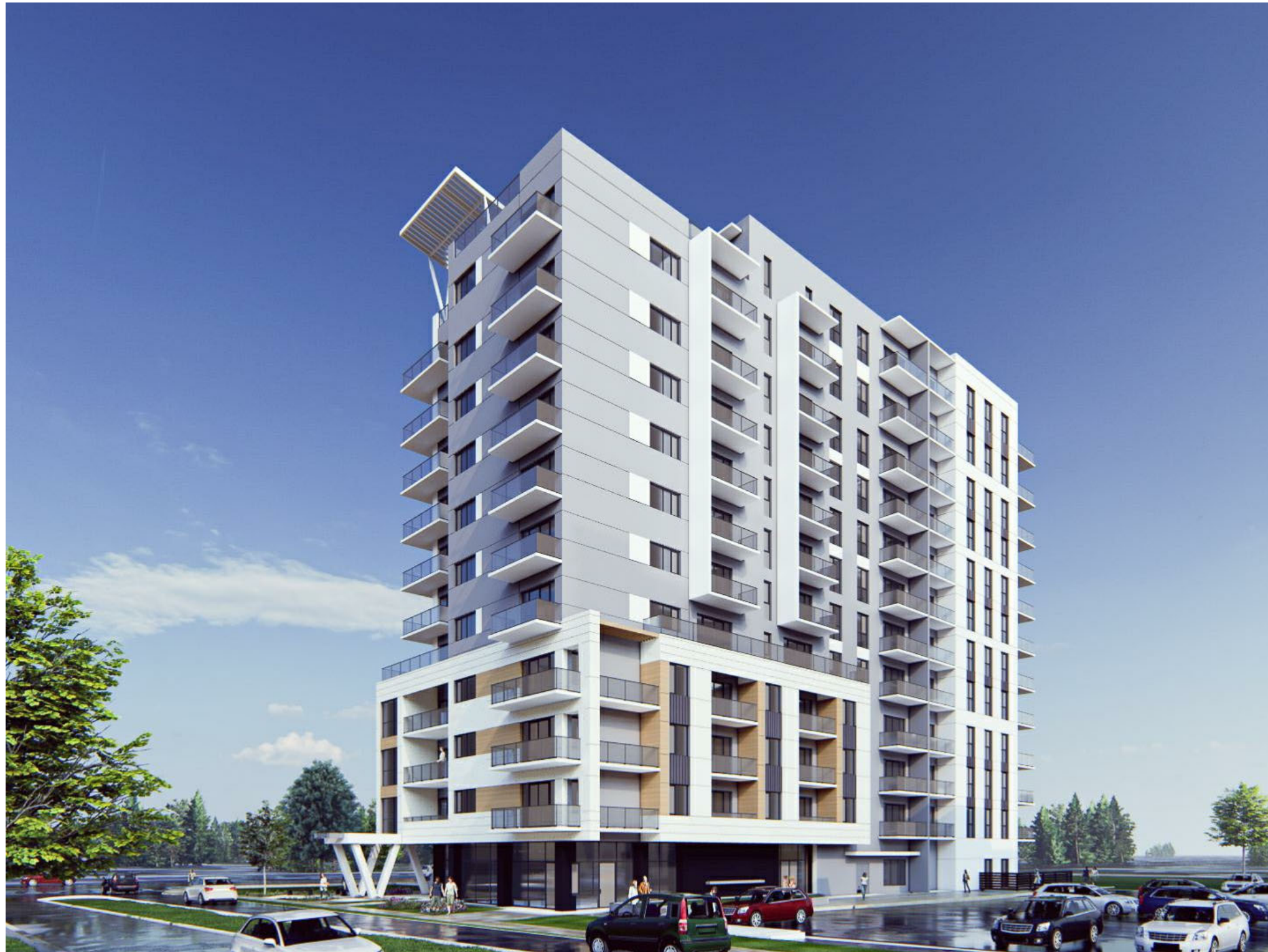
View from Yorkville St looking Northeast
