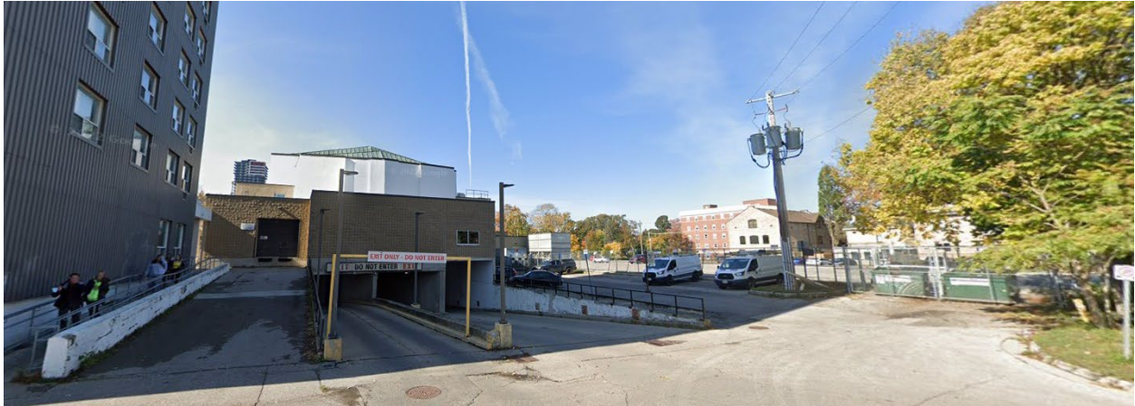
Figure 16 – Abutting residential dwelling to the east of the subject lands
