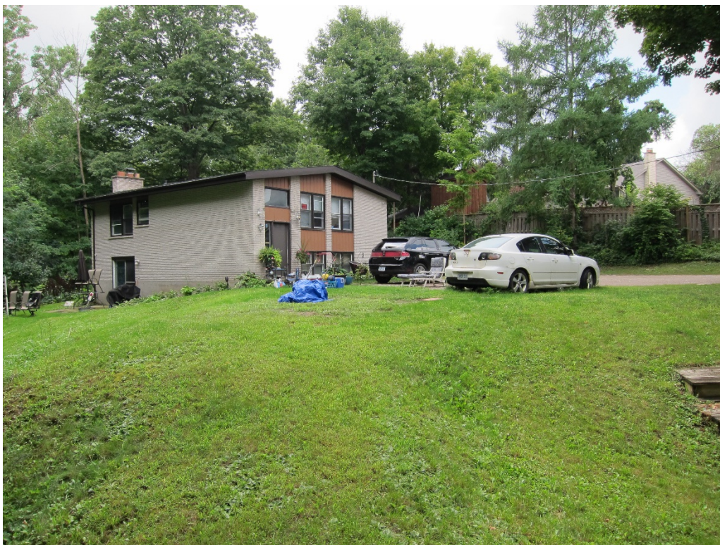
Photo No. 8. View of house and parking area looking southwest.
