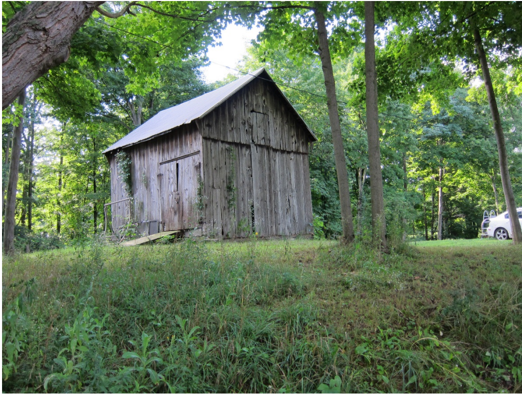
Photo No. 3. View of wood frame shed looking northeast.
