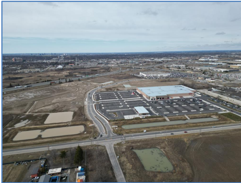
Figure 5 – Aerial view of subject lands looking north
