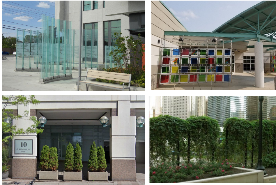
Image 10: Wind control measures for building corners
