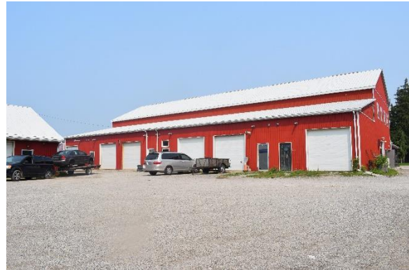
Plate 51: South elevation, looking north
