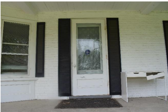
Plate 22: Main entrance door, looking south
