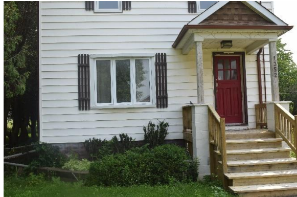
Plate 39: First storey of west elevation, looking east
