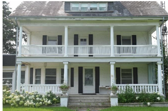
Plate 21: View of porch and second storey details, looking south
