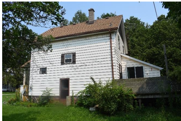
Plate 43: South elevation, looking north
