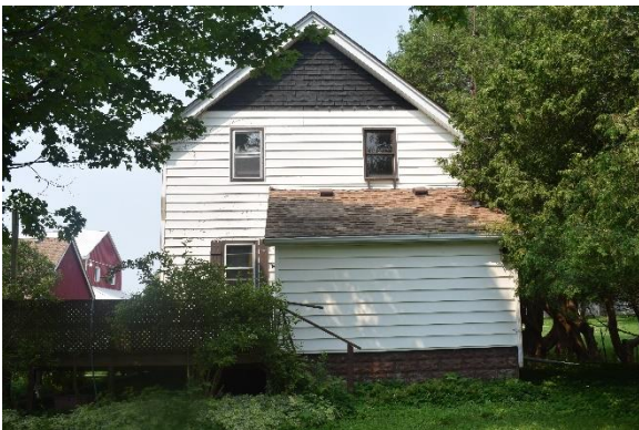
Plate 42: East elevation, looking west
