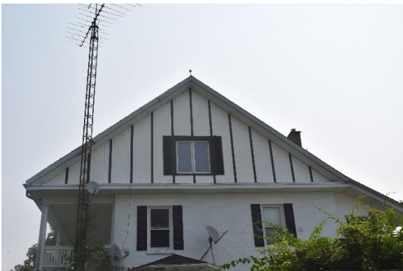
Plate 28: Second storey details, looking east
