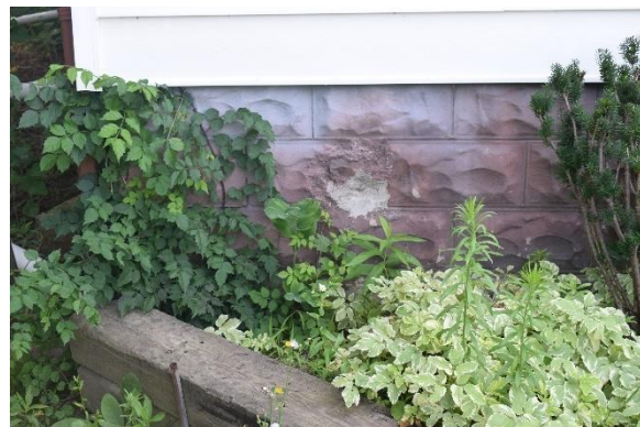
Plate 37: Foundation, looking east
