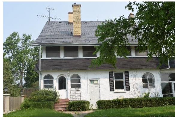
Plate 33: South elevation, looking north
