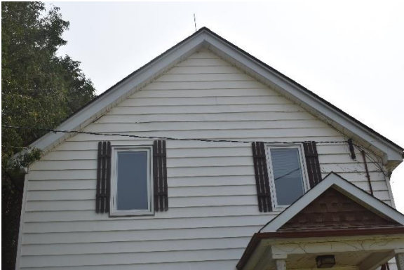
Plate 38: Second storey of west elevation, looking east
