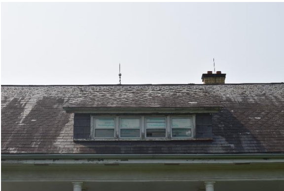
Plate 20: Shed roof dormer, looking south
