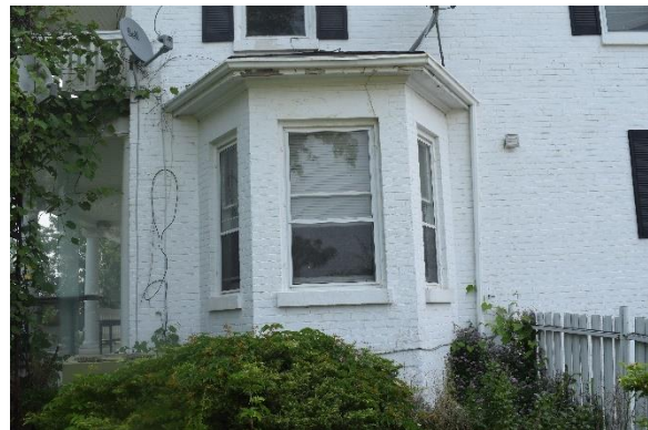
Plate 29: Bay window, looking east
