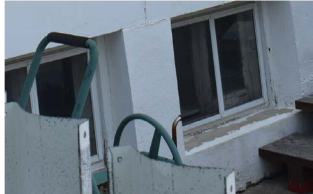
Plate 19: Concrete foundation, looking east
