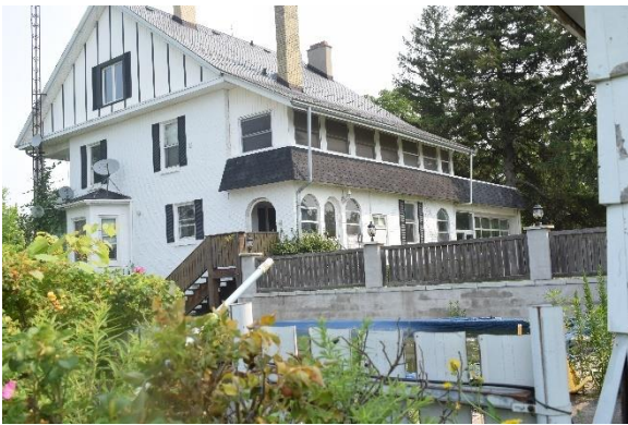
Plate 32: Looking northeast at shed roof addition
