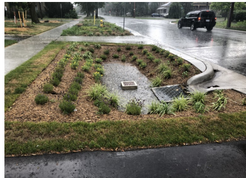
Rain gardens located along Waterloo Street
