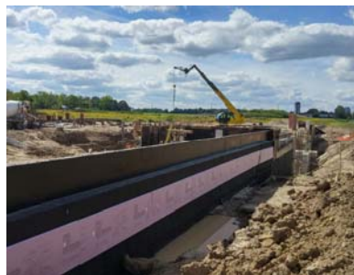
5. Foundation wall along Southdale Road
