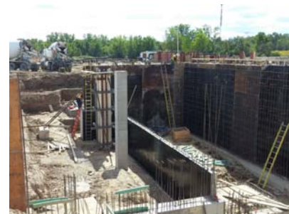
6. Excavating and construction for basement
