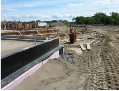
7. View towards south of site – gymnasium corner
