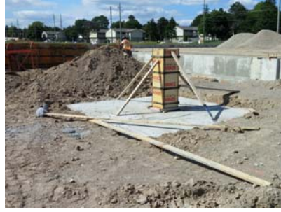
8. Pad footing – north east corner of rink
