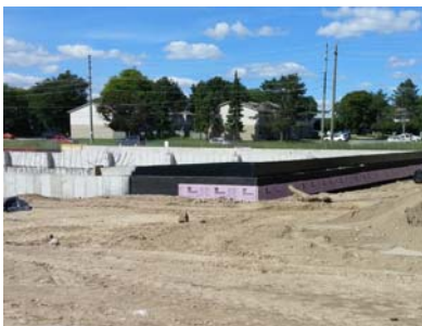
4. North view towards Southdale Road – pool corner
