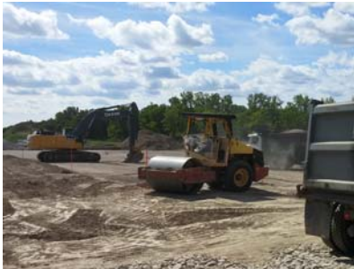
1. View towards south of site – construction of parking lot
