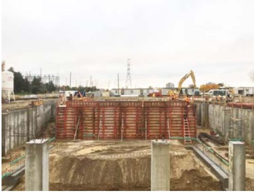
6. View of pool basin construction
