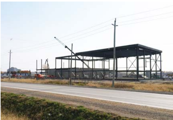
3. Gymnasium steel – northwest corner of site
