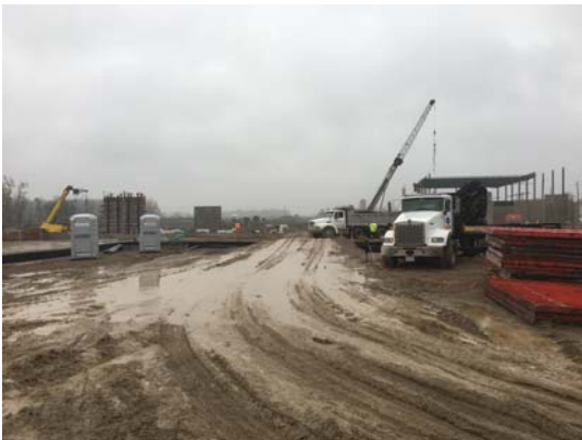
1. View of the east plaza looking west
