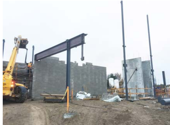
4. Masonry and bearing steel over fitness area
