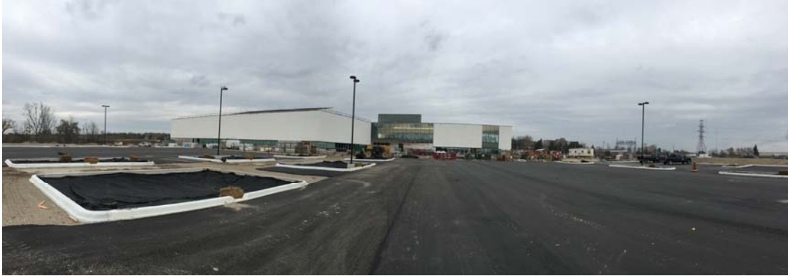
8. View from parking lot to South building entrance.
