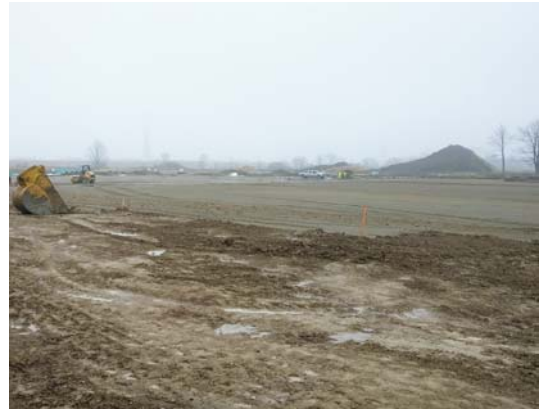
7. Parking lot taking shape.
