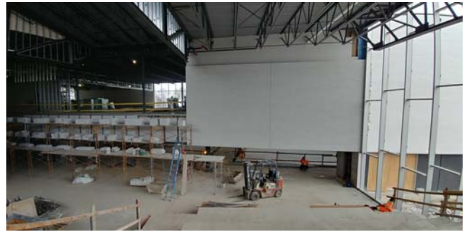
8. Interior masonry under way at base of Gathering Stair
