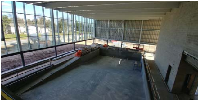
1. View from Level 2 to Aquatics Hall lap pool
