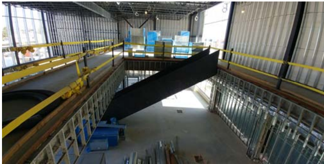
7. View of Library Mezzanine east
