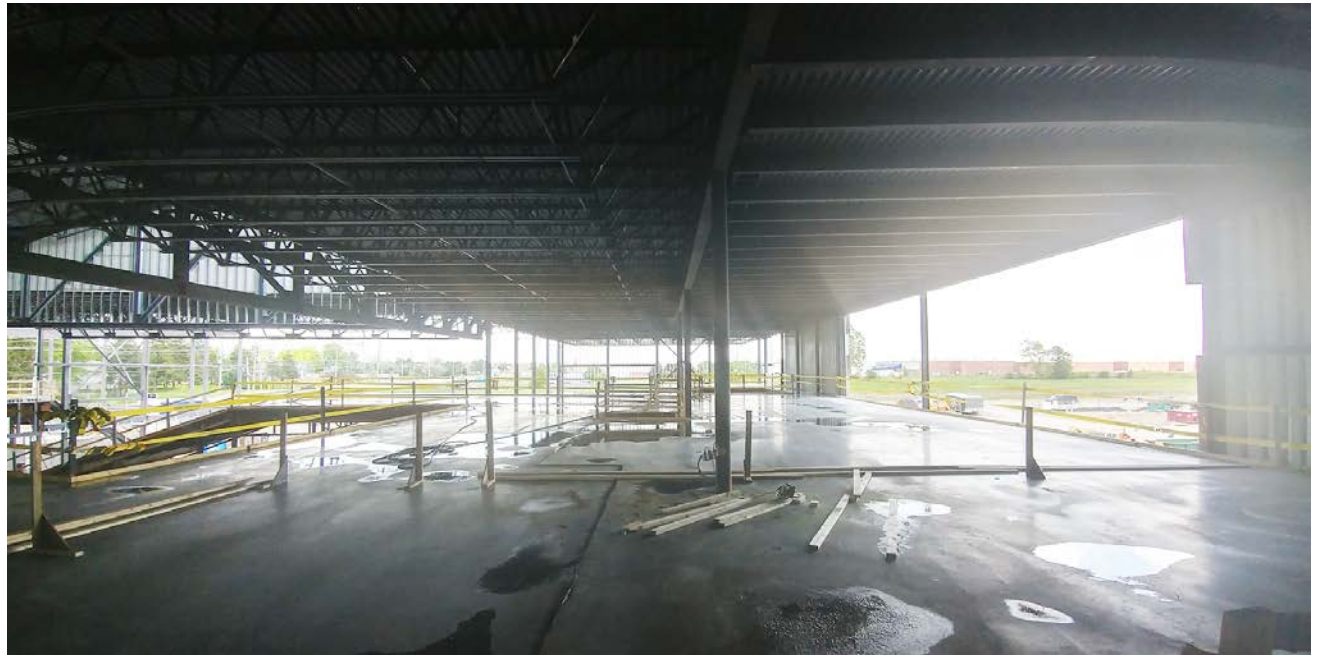
5. Second floor multipurpose wing area looking east.
