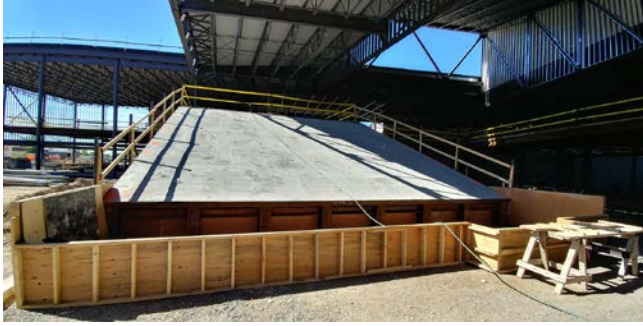
1. View of gathering stair form work looking south.
