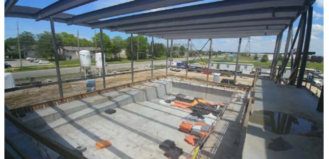
2. Lap pool and structural steel. Accessible ramp in the background.
