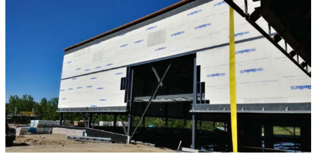
6. Rink 2 east wall cladding installation in progress.
