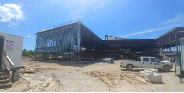
6. East wall of library steel stud work.
