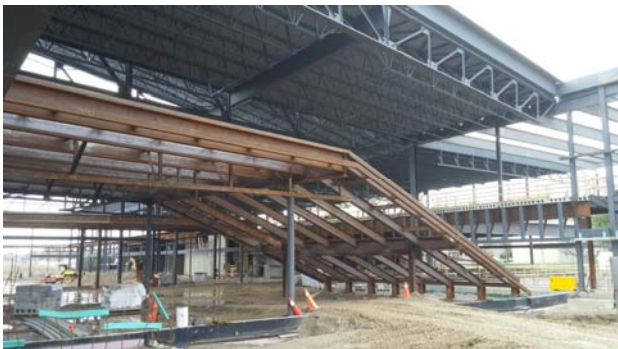
3. Structural steel – stairs in the Gathering Area
