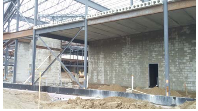
6. Core slab in mechanical area at west side of Rink 2
