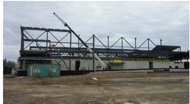
2. View looking North of Rink 2 steel.
