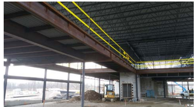
4. Steel for interior of Library looking west.
