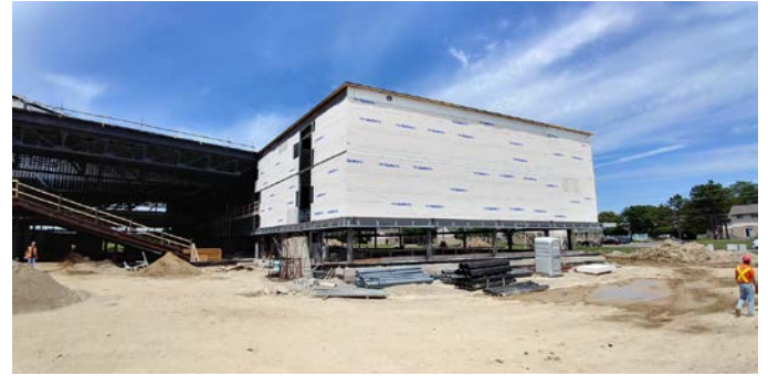
6. Pool wing exterior cladding in progress.
