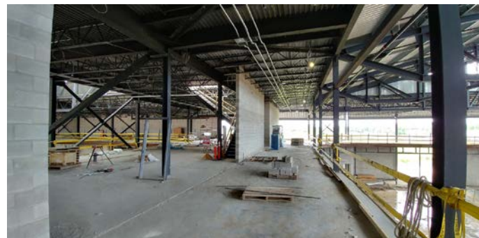
4. Second floor Multi-Purpose Room wing masonry.
