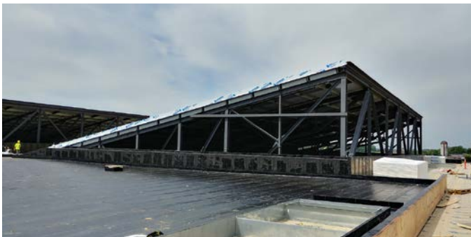
1. View of arena skylights roofing ongoing.
