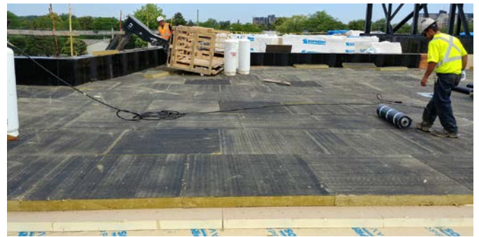
2. Building roofing continuation.
