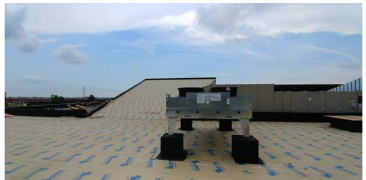
10. Roof installation in progress.
