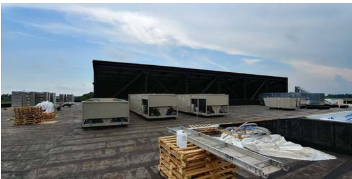
9. Roof top units installation in progress.
