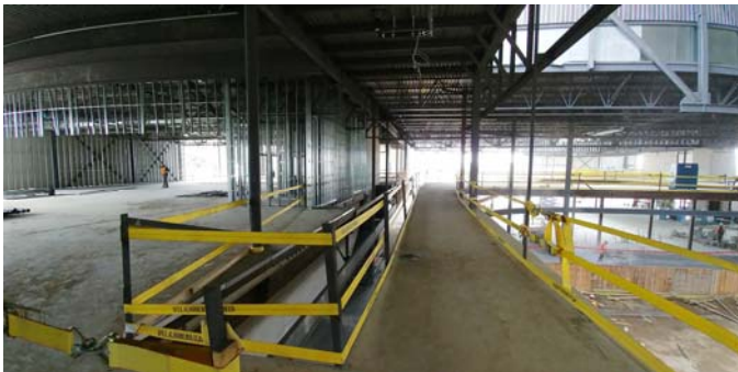
1. View of the walking loop looking east.
