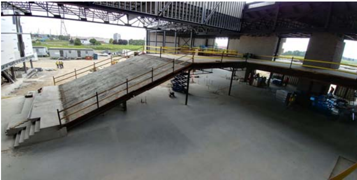
5. Concrete work for the Gathering Stair in progress.
