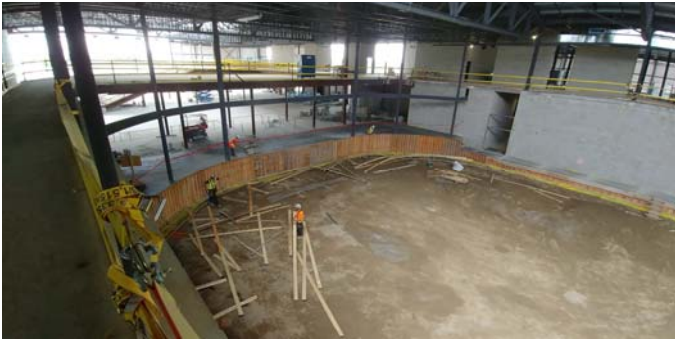
3. Rink 1 concrete work in progress.
