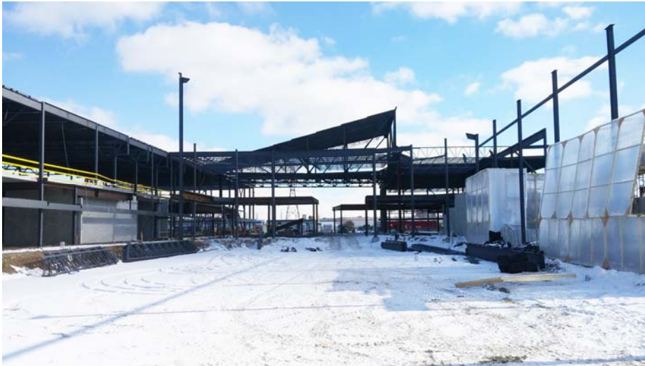
1. View looking east from Rink to Gathering Space Skylight.
