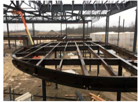
5. Structural steel for the Level 2 Walking Loop
