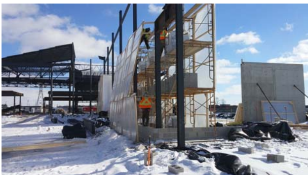
2. Arena Change Rooms – masonry
