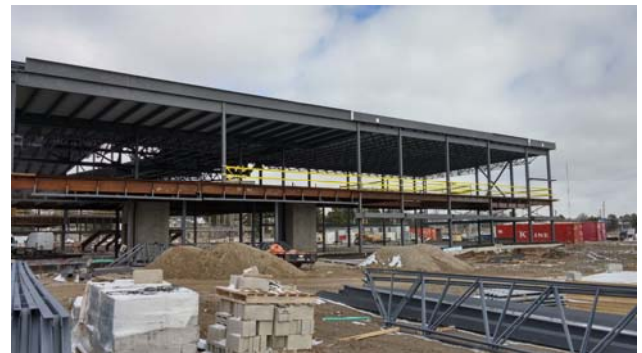
3. South side of Library, north view.
