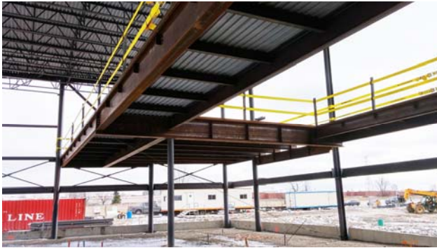
4. Library second floor stair opening and connection to upper space
