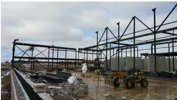
2. North rink structural steel
