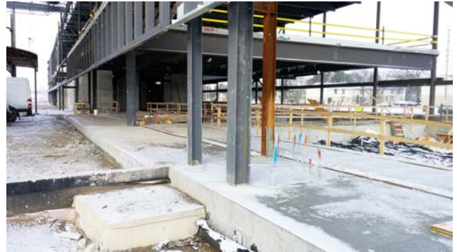
5. Structural concrete floor over basement
